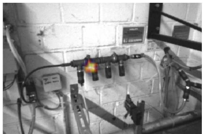
Leakage at the separator
